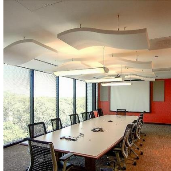
Lighting and acoustic clouds battle for space, making for a lot of clutter in the ceiling
