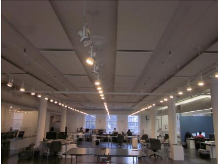
Approximately one kajillion track heads are used to provide general illumination to make room for acoustic panels
