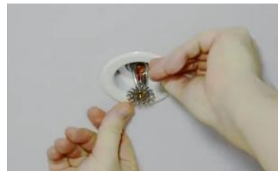
2. Press the escutcheon into place until secured
