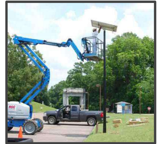
Commissioning and aiming
