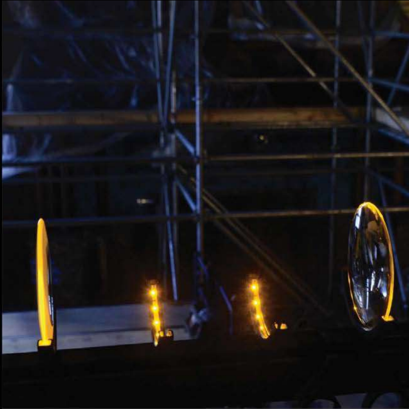
MOCK-UP LIGHT SOURCE 3/8" WIDE LED STRIP LIGHT RECESSED IN FRAME
