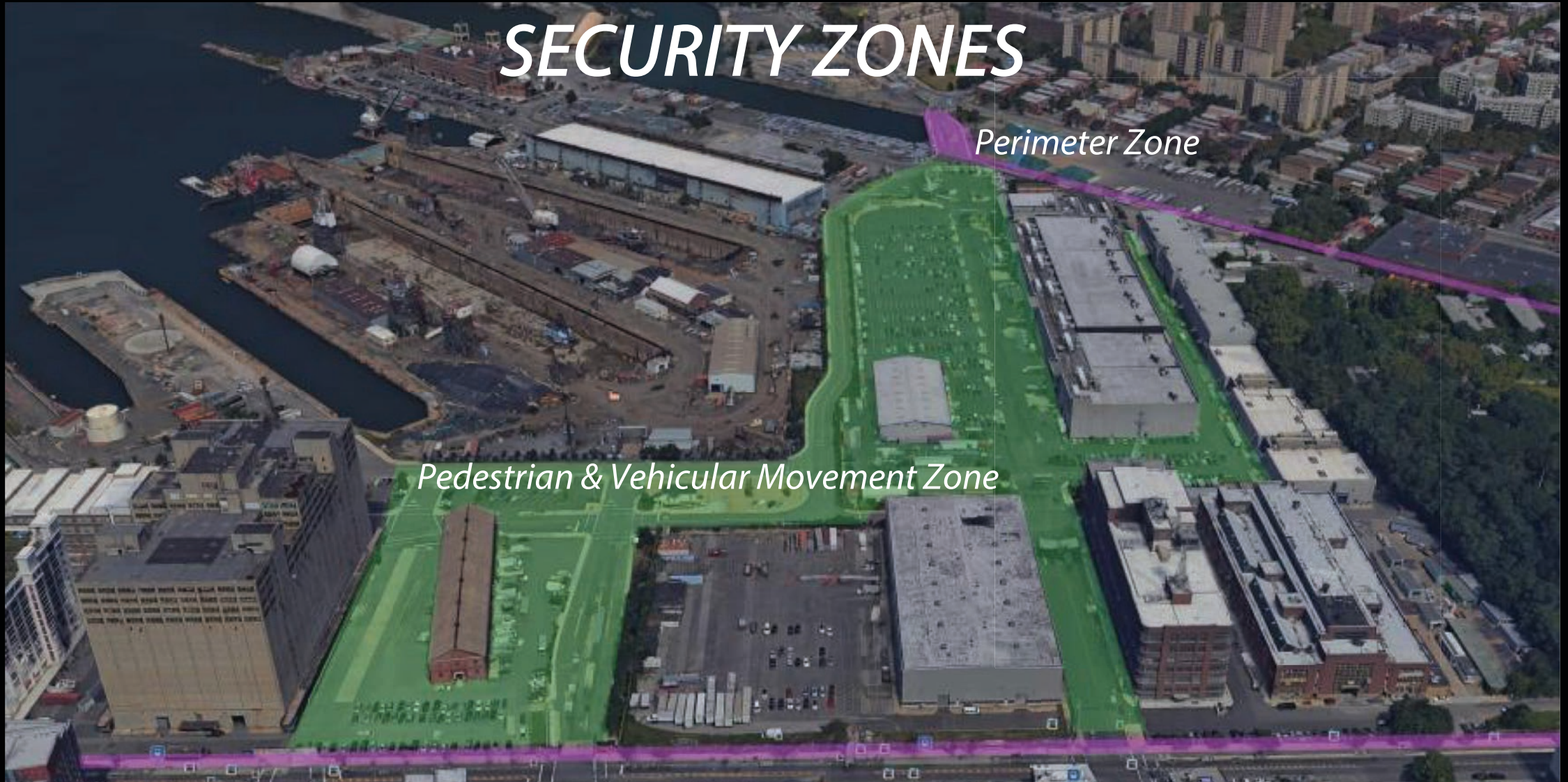
IES G-1-16 Guidelines for Security Lighting for People, Property and Critical Infrastructure Image: Google Earth – Brooklyn Navy Yard, Brooklyn NY
