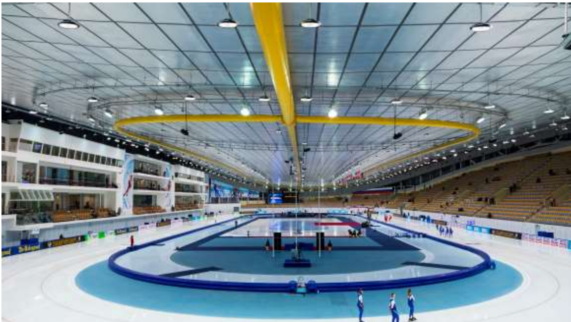
Whiz 2.0 Example Installation
