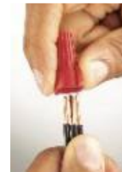
Line Voltage Connections
