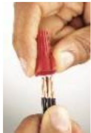
Line Voltage Connections
