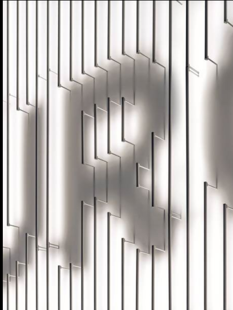
A DETAIL SHOWING THE CUSTOM STANDOFFS THAT DOUBLE AS DISCREET WIREWAYS.
